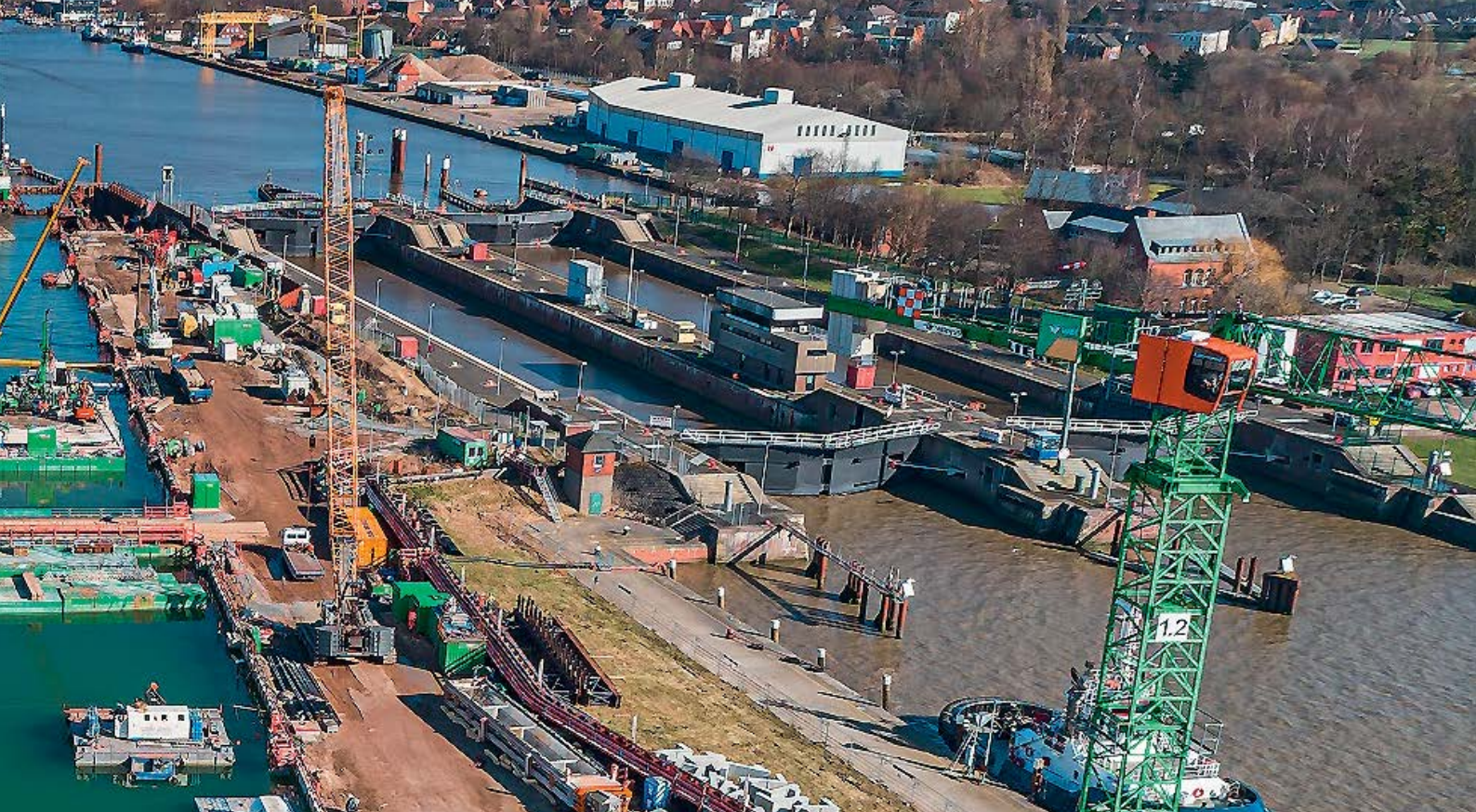
Construction of the fifth lock chamber at Brunsbüttel
