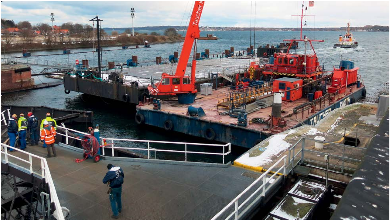
Replacement of a sliding gate at the Brunsbüttel lock
