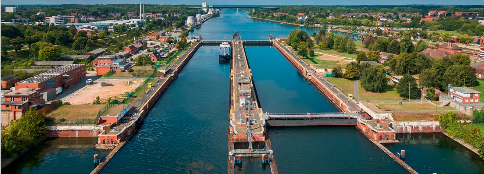
Lock installation at Kiel-Holtenau
