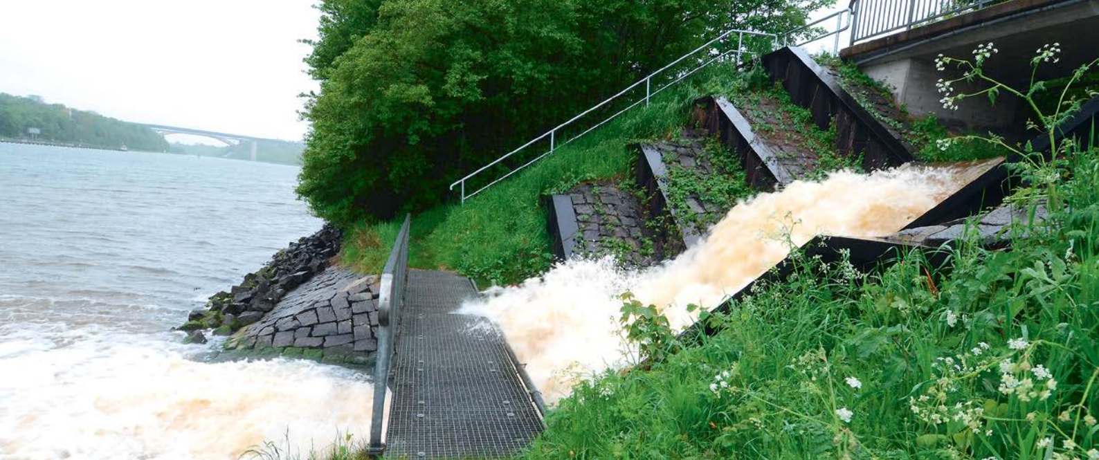
Inlet structure near Projensdorf
