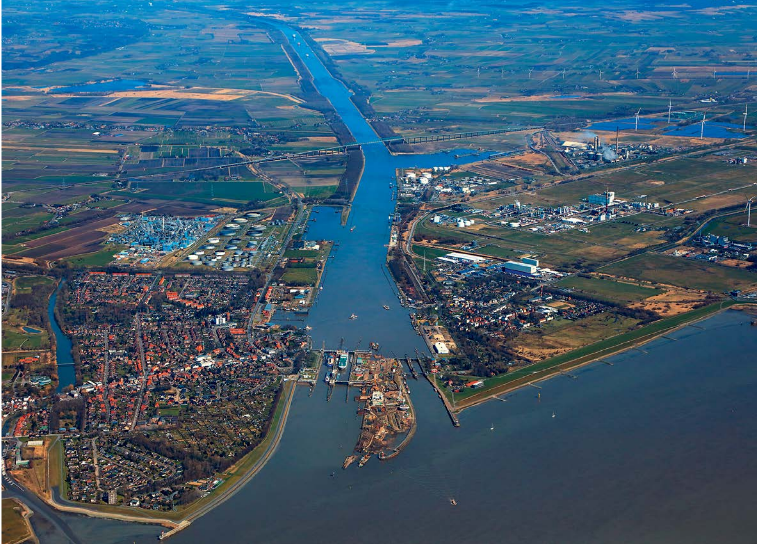
Locks at Brunsbüttel
